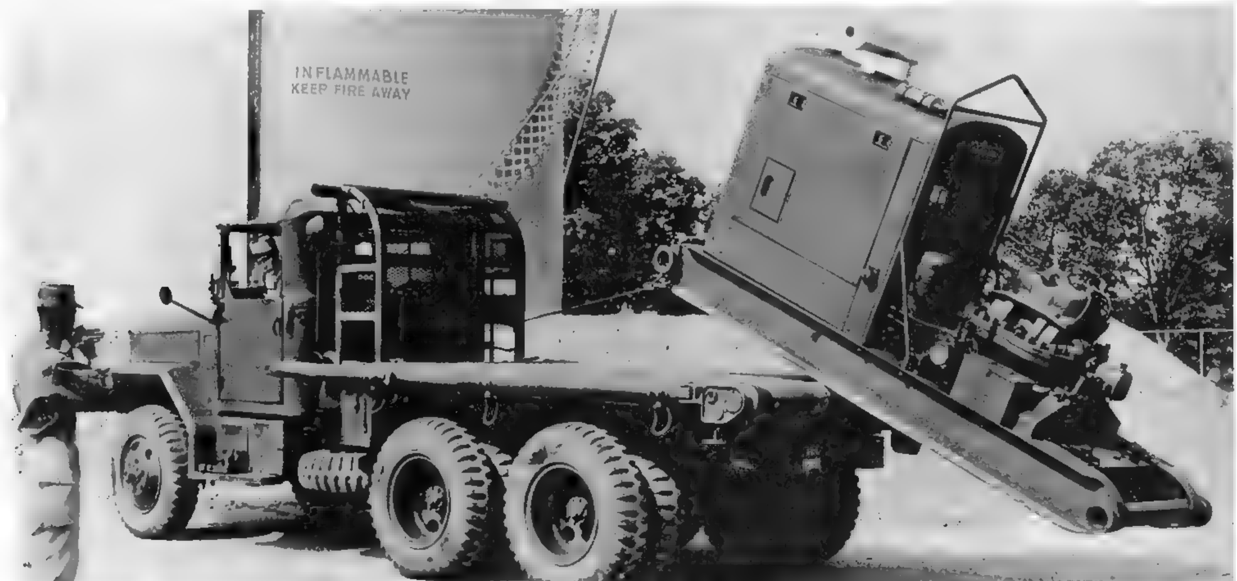
This truck has a pipeline construction conversion kit installed. It is unloading a pumping unit here. (Photo courtesy of United States Army Engineer School History Office)
